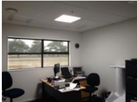
Solar Tube @ DC Office & Spare parts Warehouse
